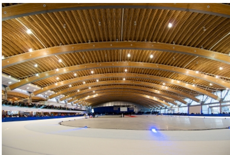
Fig. 1.1: Olympic oval, Richmond, Canada
